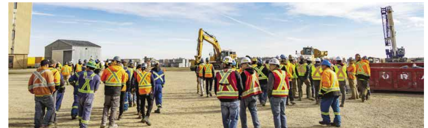
Buffalo Pound Water Treatment Plant Site
