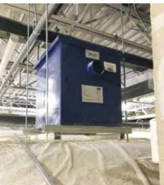
Grease trap. This is hung in the crawl space located just off the basement hallway, beneath the kitchen.
