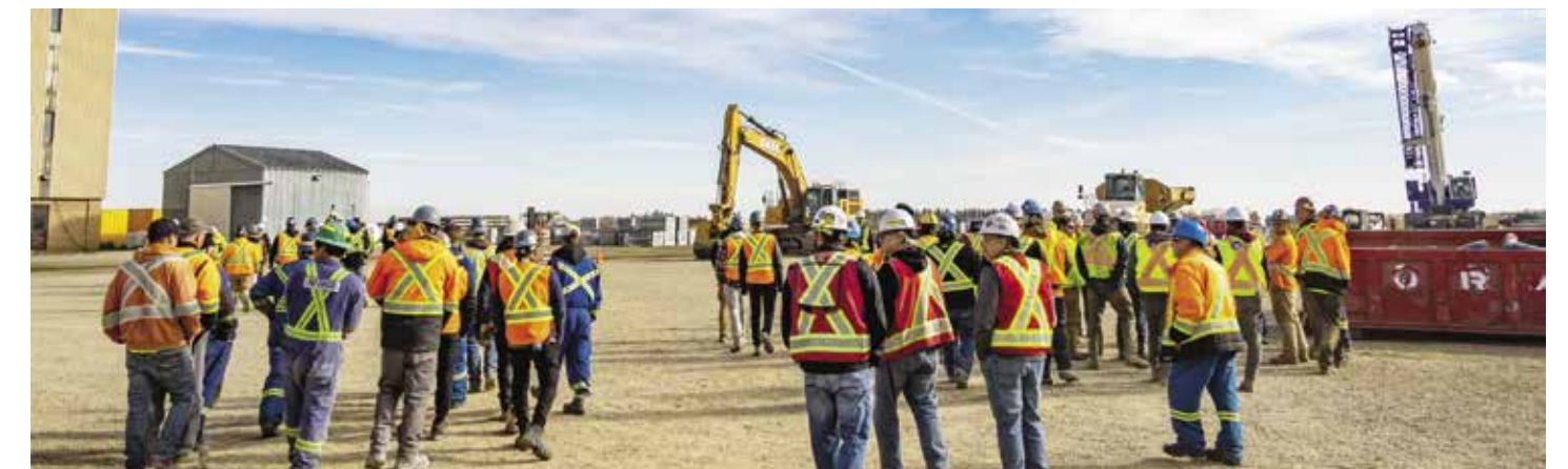
Buffalo Pound Water Treatment Plant Site
